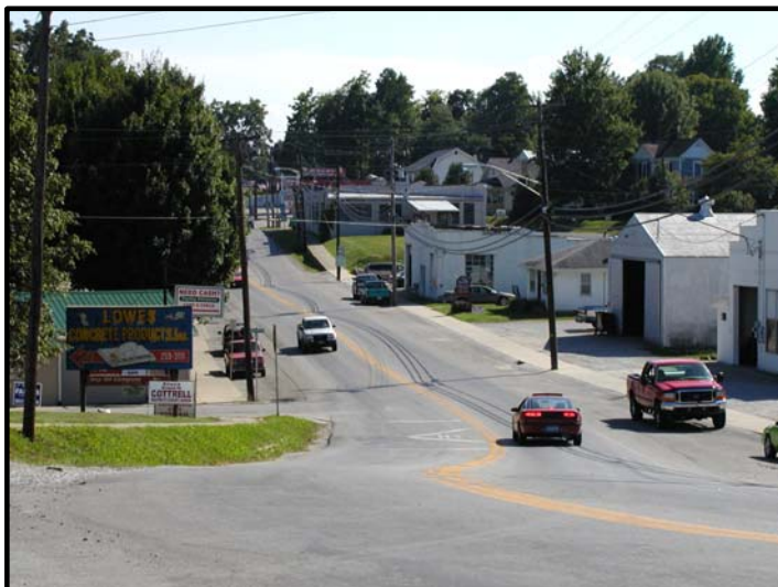
Sidewalks in Good Condition but Close to Roadway
